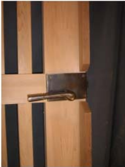
Illustrating the alignment of the strike plate to the latch bar. (In humid salty regions such as Miami, the bronze can develop a white film. This is easily cleaned with water.)
