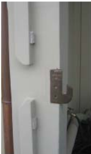
Showing the configuration of the gate stops to clear the Euro plate. Note the Strike is mortised flush to the post
