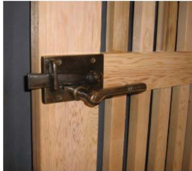
The typical latch bar plate. The plates do not always align themselves with the mid-rail of the gate.
