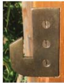
Typical strike plate mortised flush to the post or jamb
