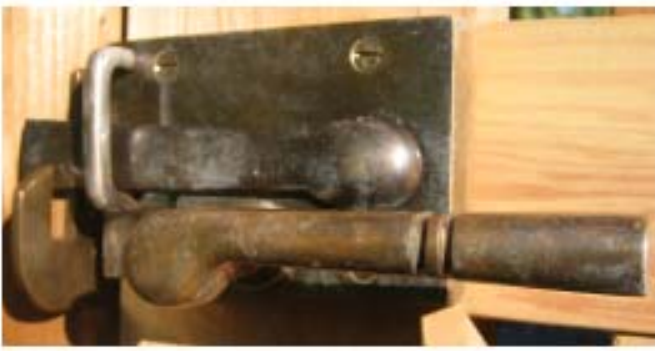
Illustrating the alignment of the strike plate to the latch bar. (In humid salty regions such as Miami, the bronze can develop a white film. This is easily cleaned with water.)
